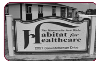
Signage and new Habitat for Healthcare building
