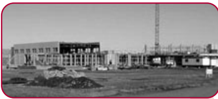
Construction on the new Cypress Regional Hospital Underway
